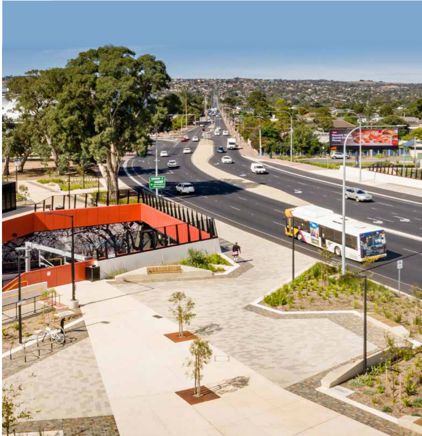
Figure 3. Oaklands Crossing, Adelaide
