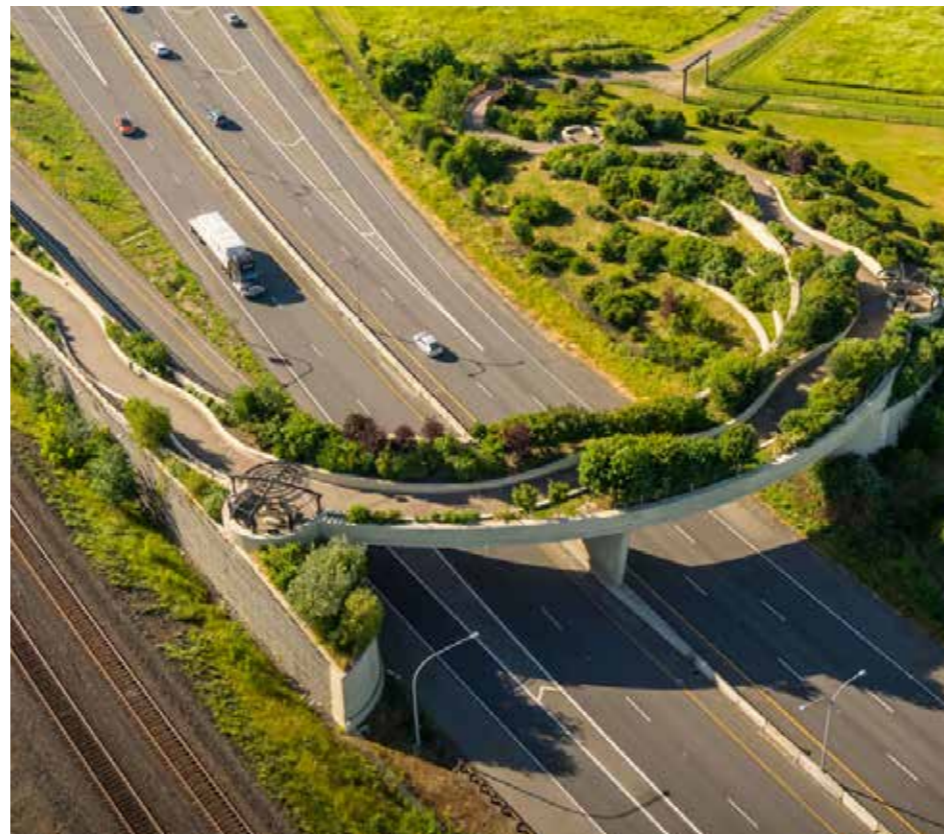
Figure 55. Vancouver Land Bridge, Washington, USA. The bridge utilises a raised planter design to hold appropriate depth and profile of growing medium and support healthy planting.
