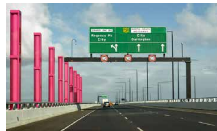
Figure 81. Darlington Upgrade Project (above) and South Road Superway (below), Adelaide. Gantries consolidate signage and associated infrastructure to minimise the need for additional overhead structures.
