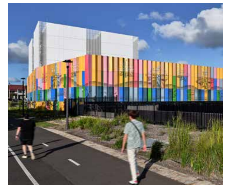
Figure 70. WestConnex Tunnel Support Facility, Sydney. The tunnel portal design and creative elements achieve a distinct sense of identity whilst also providing screening for ventilation facility above.
