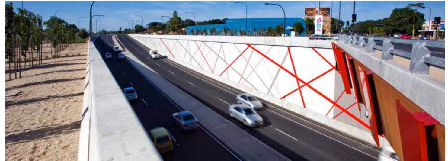
Figure 46. Gallipoli Underpass, Adelaide. Creative treatments on retaining walls enhance user experience and panel fixings and structural elements are concealed from view.
