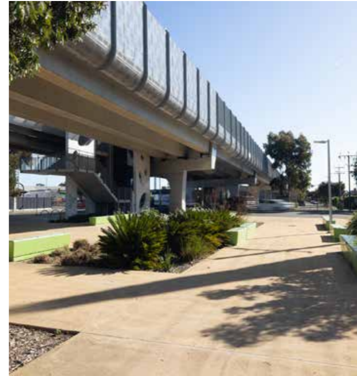
Figure 29. South Road Tram Overpass, Everard Park
