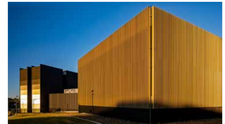
Figure 69. WestConnex M5 MOC3 Buildings, Sydney. The architectural treatments to buildings achieve a well considered outcome that visually minimises bulk and is also coordinated with the tunnel portal treatments.
