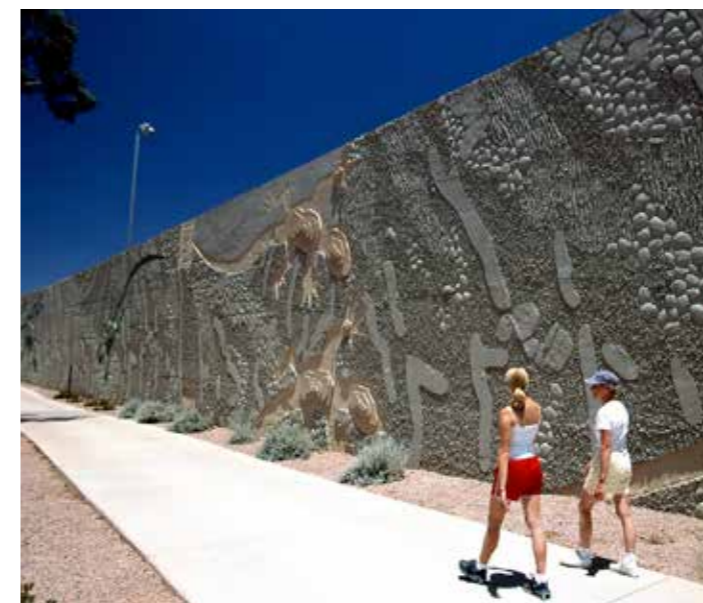
Figure 73. Pima Freeway, Scottsdale, Arizona USA. Incorporates culturally relevant, creative elements that addresses both sides of the wall and are also repeated within the wider landscape design for the road.
