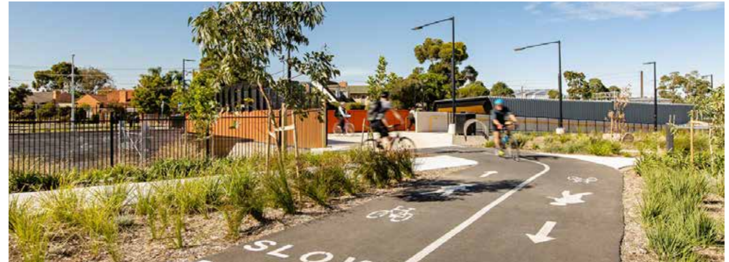
Figure 87. Oaklands Crossing, Adelaide. Active travel paths are enhanced with landscaping and have a smooth, even surface free from obstructions.
