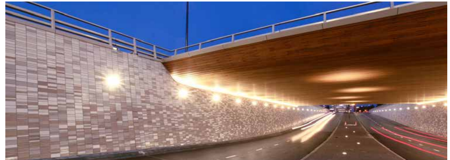
Figure 47. Bio Science Park, Netherlands. Texture and patterning of the walls visually minimise the impact of their height. Timber treatments to the underside of the bridge provide an attractive and memorable treatment that conceals structural elements.
