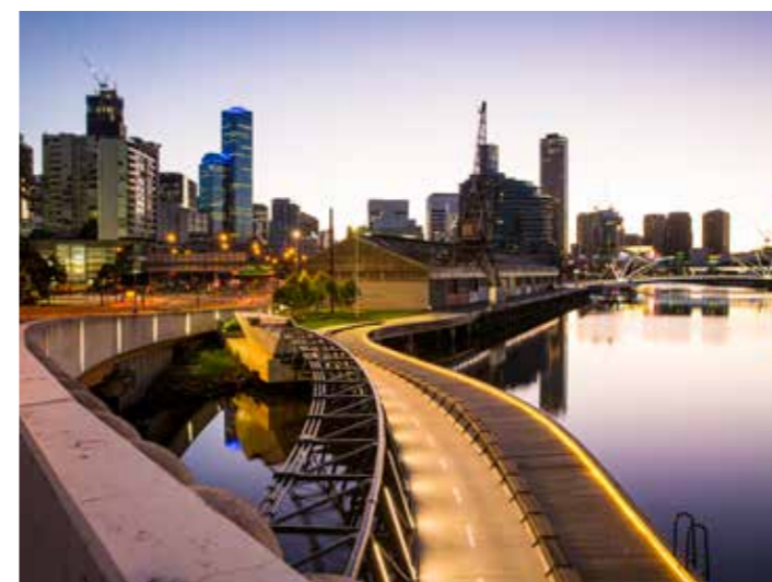
Figure 93. Jim Stynes Bridge, Melbourne. Creative use of feature lighting that is integrated with bridge and public realm elements.
