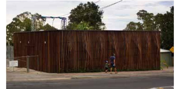
Figure 68. Burnside Substation, Adelaide. Creative design of electricity substation screen assists in concealing unsightly elements.
