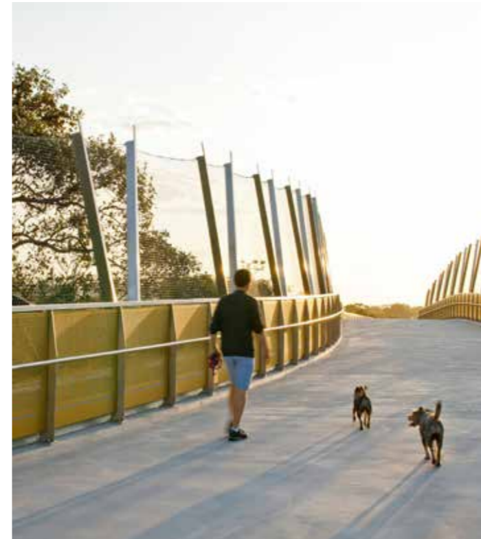
Figure 75. Albert 'Tibby' Cotter Walkway, Sydney. Throw screens use a tensile mesh that is visually permeable offering good surveillance and views for users whilst being strong and lightweight.
