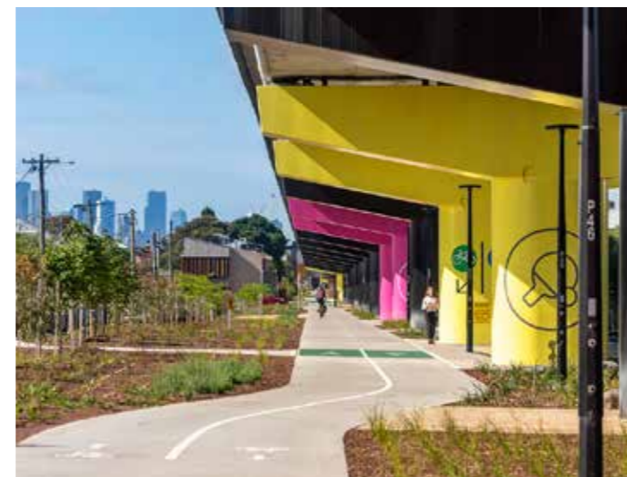
Figure 88. Bell to Moreland Level Crossing Removal Project, Melbourne. Use of colour assists with wayfinding and orientation.
