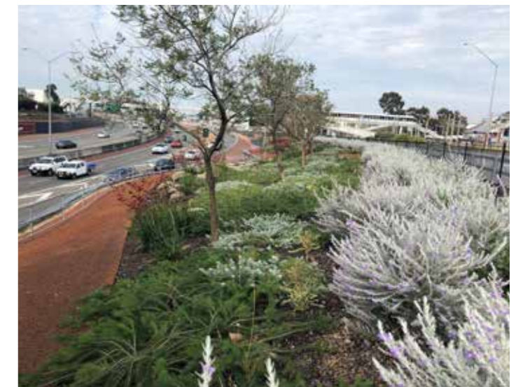
Figure 100. Graham Farmer Freeway, Perth. Landscape design allows for safe maintenance access.
