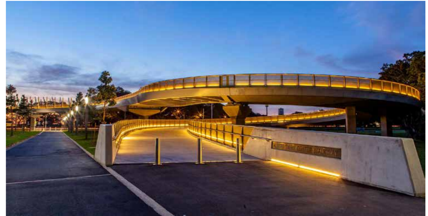
Figure 50. Albert 'Tibby' Cotter Walkway, Sydney. The design has structurally expressive sculptural form with lighting that gives prominence at night and bollards that are integrated with the design.
