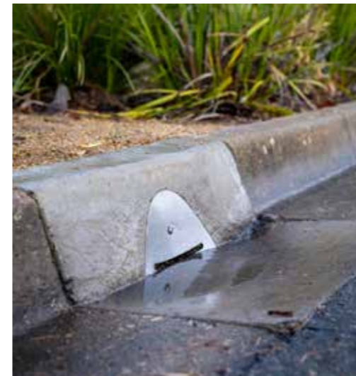
Figure 112. Tree net inlet allows for innovative storm water irrigation of adjacent tree pits and planting.
