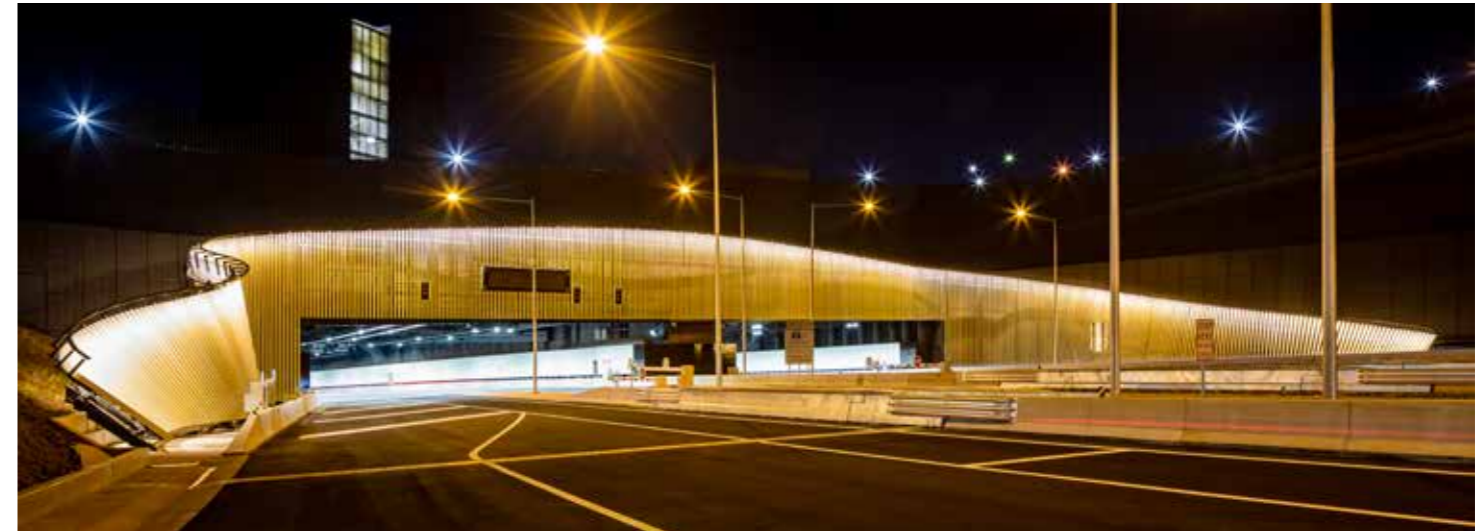
Figure 91. WestConnex M8 Tunnel Portal, Sydney. Lighting is used to highlight architectural features of the portal design as part of the project's distinct identity.
