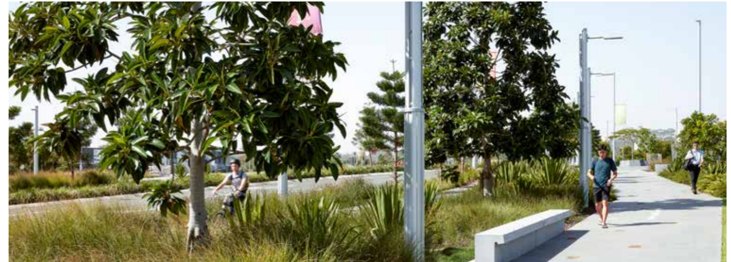
Figure 83. Aerodrome Road Intersection, Maroochydore. Wide verges provide ample space for separated pedestrian and cyclist paths. Places to rest and stop are surrounded by planting and trees for shade. Street furniture including light poles are located to avoid being obstructions and reduce clutter.
