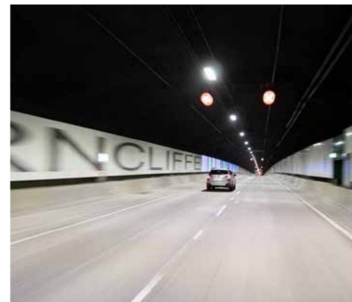
Figure 64. WestConnex M8 Sydney, Sydney. Large distinctive lettering enables an awareness of location whilst underground. The light coloured panels on the walls with a dark roof increases the sense of spaciousness and calm.
