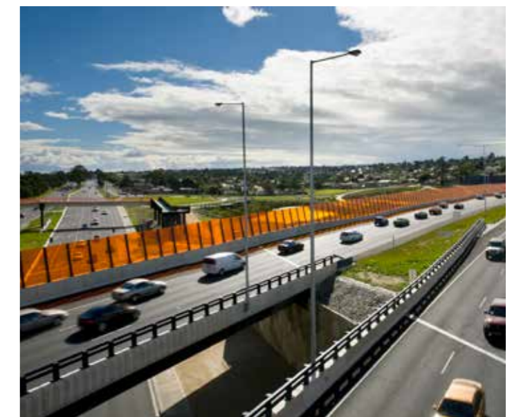
Figure 74. Eastlink Freeway, Melbourne. The noise barrier is incorporated into the design of the bridge structure and angled away from the road for improved visual outcomes.
