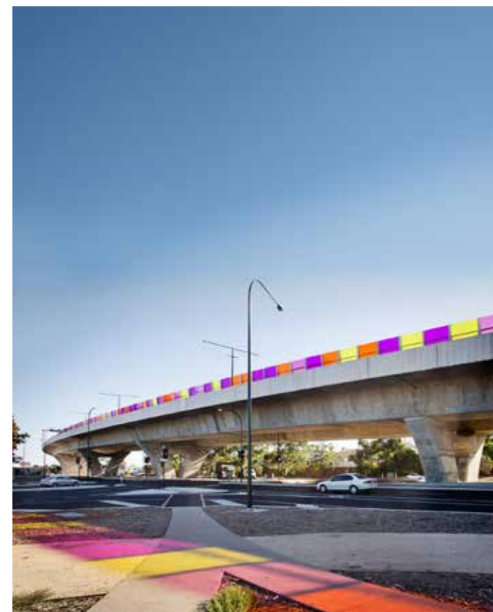
Figure 76. South Road Superway, Adelaide. The design of the throw screens on the bridge adopt consistent repeatable patterns that create visual interest at ground level.
