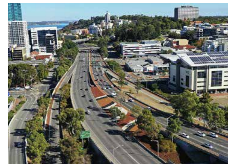
Figure 101. Mitchell Freeway, Perth. Planted medians improve the sense of 'green', reduces heat island effects and provide culturally relevant, creative design responses.
