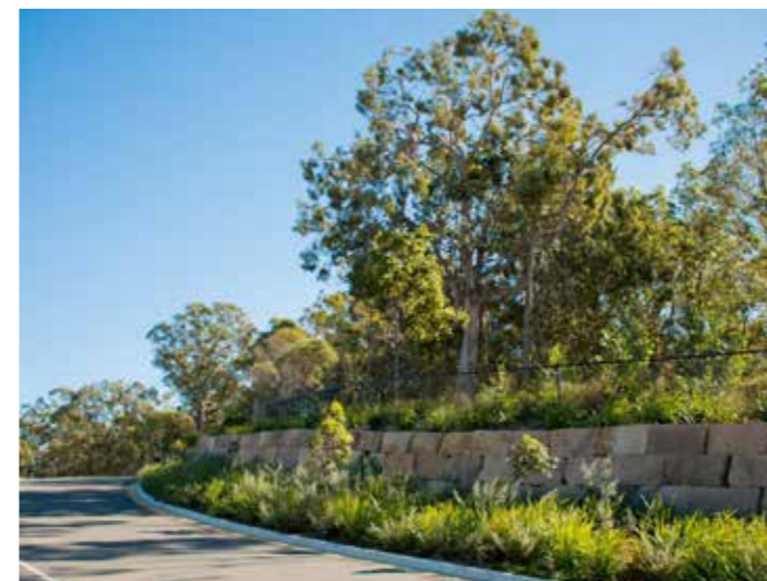
Figure 107. Minnipi Parklands, Brisbane. Vegetation has been used to soften the appearance of retaining walls.
