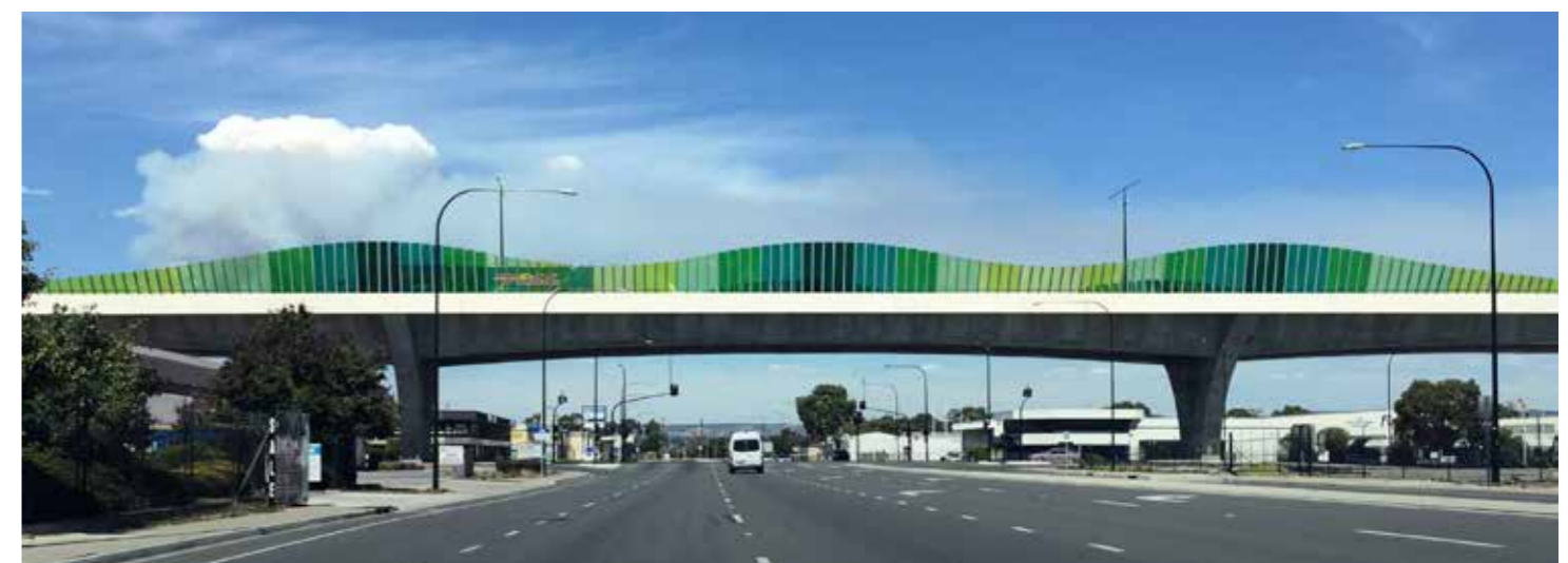
Figure 45. South Road Superway, Adelaide. The design is structurally expressive with well proportioned superstructure and a large span to minimise piers and maximise the sense of openness.
