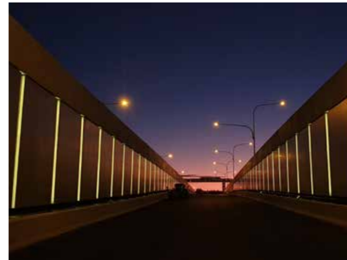
Figure 92. WestConnex M8 Kingsgrove Dives, Sydney. Vertical light bars within lowered road walls create a special effect for road users at night.
