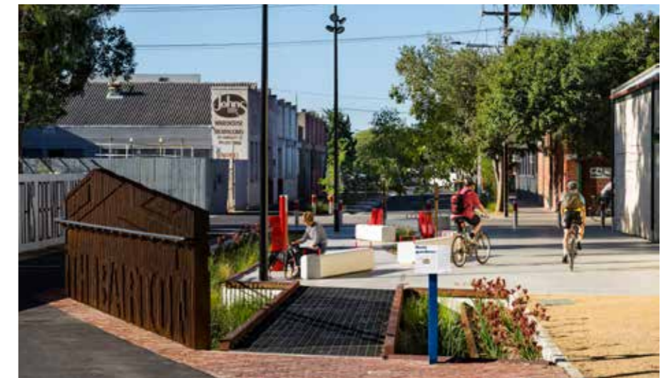
Figure 113. Holland Street, Thebarton. Passive irrigation techniques drain runoff from streets into planting beds and rain gardens are an integrated feature of the public realm.
