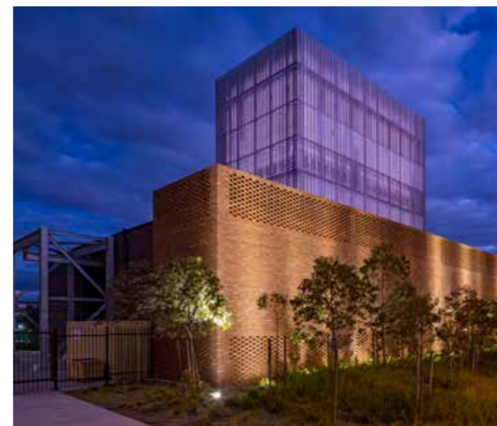
Figure 67. WestConnex Parramatta Road Ventilation Facility, Sydney. A 9m high translucent polycarbonate wall provides a simple, high-quality architectural treatment that becomes an interesting feature at night.
