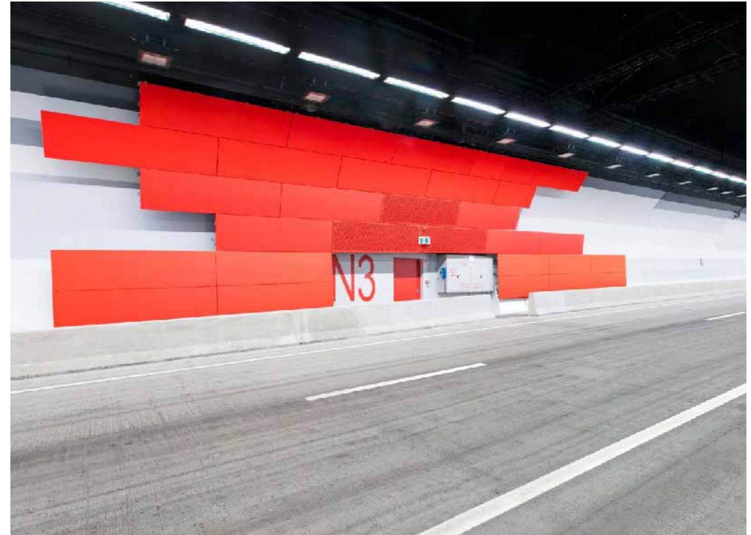
Figure 63. St Helena Tunnel, Byron Bay. Creative treatments around emergency access points help to achieve visual variety within the tunnel.
