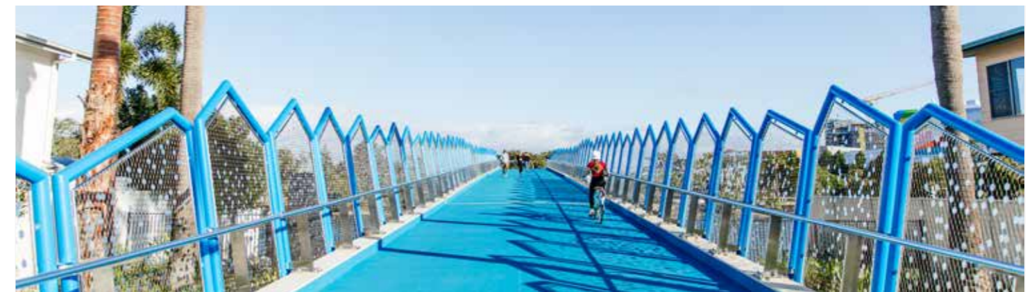
Figure 51. HOTA Bridge, Gold Coast. The bridge provides unique local experience with culturally significant place specific creative elements and great views.
