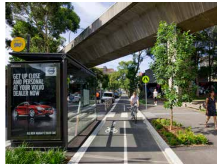
Figure 89. Bourke Street Cycleway, Sydney. Cycle paths have been designed to be integrated with bus stops to avoid pedestrian conflicts.
