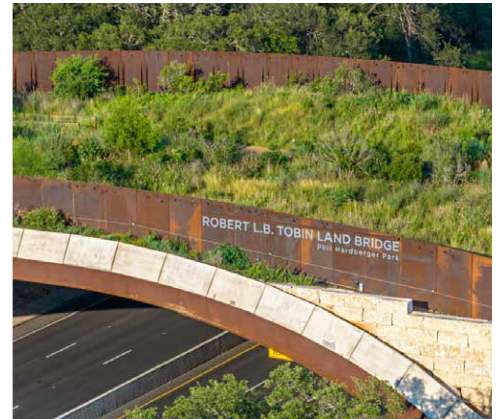
Figure 57. Robert Tobin Land Bridge, San Antonio, USA. This wildlife crossing over a major arterial road works to extend biodiversity for both wildlife and pedestrians.
