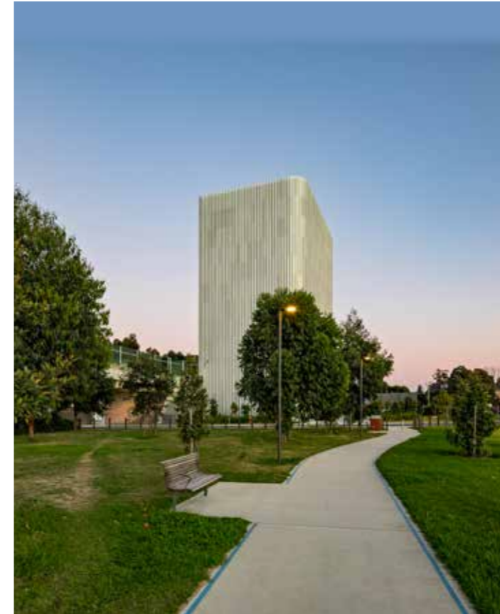
Figure 66. WestConnex M8 Ventilation facility, Sydney. Planting surrounding the ventilation structure will eventually grow to soften it from surrounding views.
