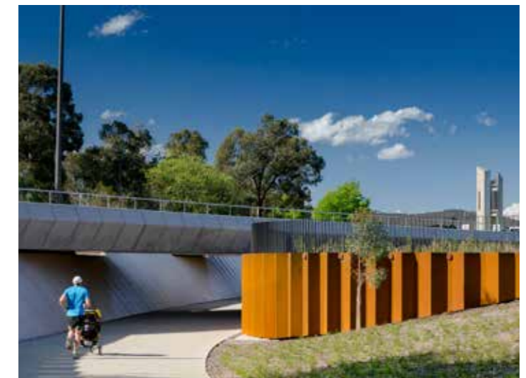
Figure 49. Bowen Place Crossing, Canberra. Feature design elements such as folded oxidised steel retaining walls and planting are used at key locations to enhance user experience.
