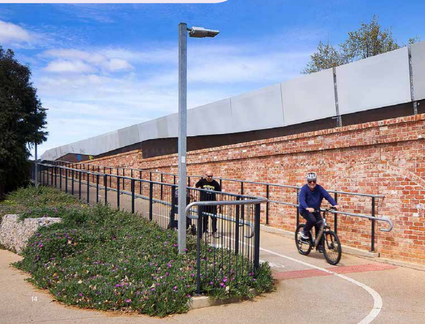
Figure 10. Torrens Road to River Torrens (T2T) Project, Adelaide
