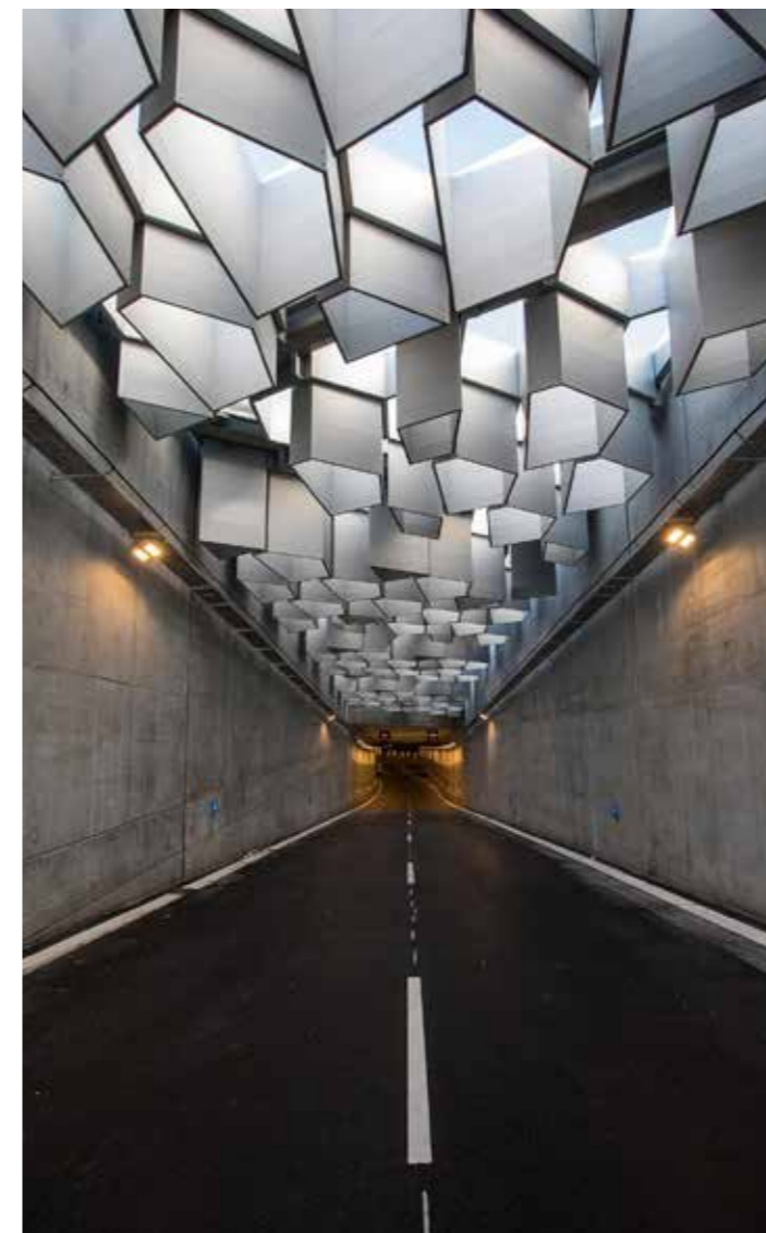
Figure 60. Nordhavn Tunnel, Copenhagen, Denmark. Distinct architectural shading devices provide a transition zone between artificial and natural light.
