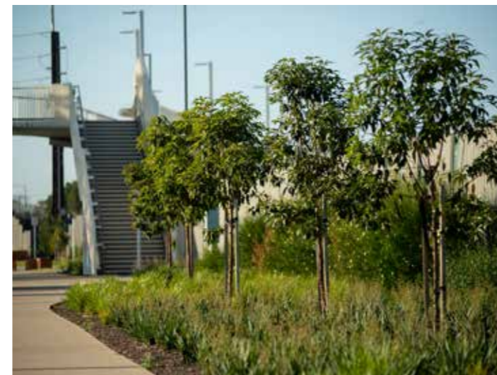
Figure 108. Regency Road to Pym Street (R2P) Project, Adelaide. Vegetation is used as a screen and landscape buffer whilst still maintaining CPTED principles.
