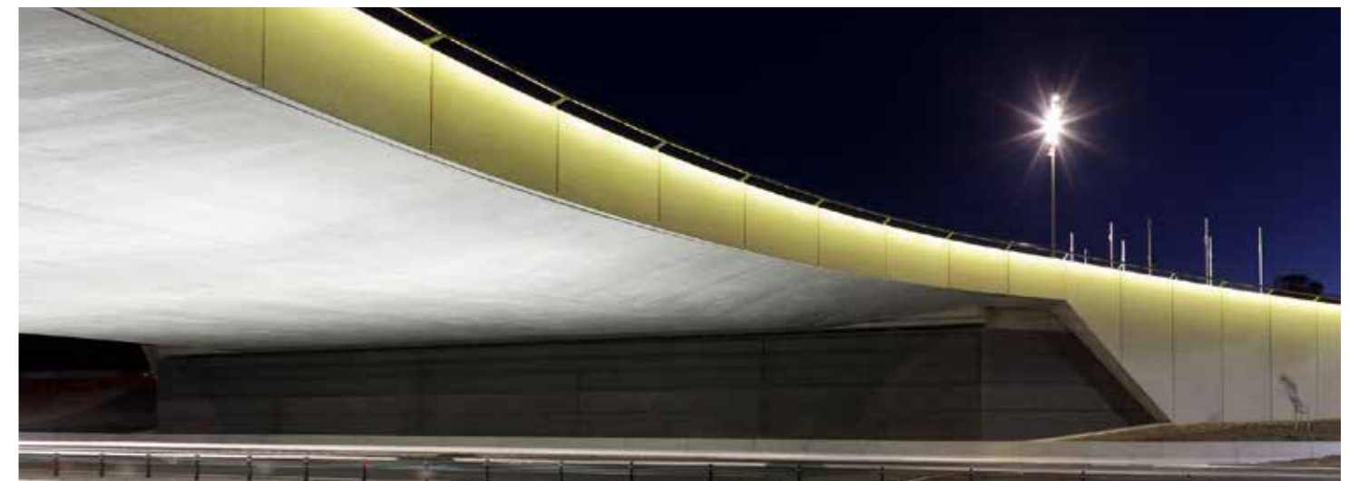
Figure 44. Kings Avenue Overpass, Canberra. Soffits are designed to conceal unsightly elements and parapets are free from visual clutter.
