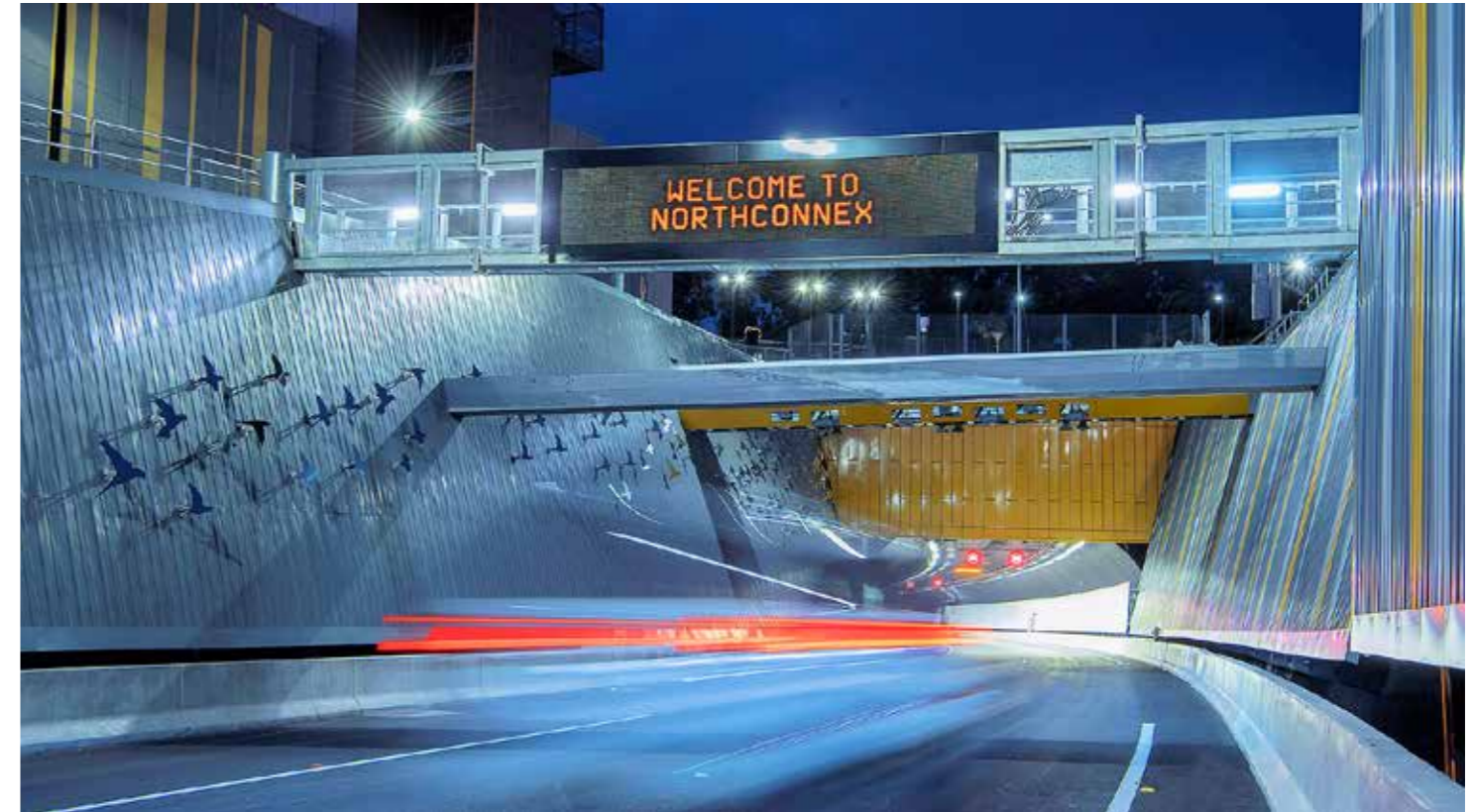
Figure 80. Northconnex, Sydney. The design successfully avoids locating signage on tunnel portal leaving the creative elements free from visual clutter.
