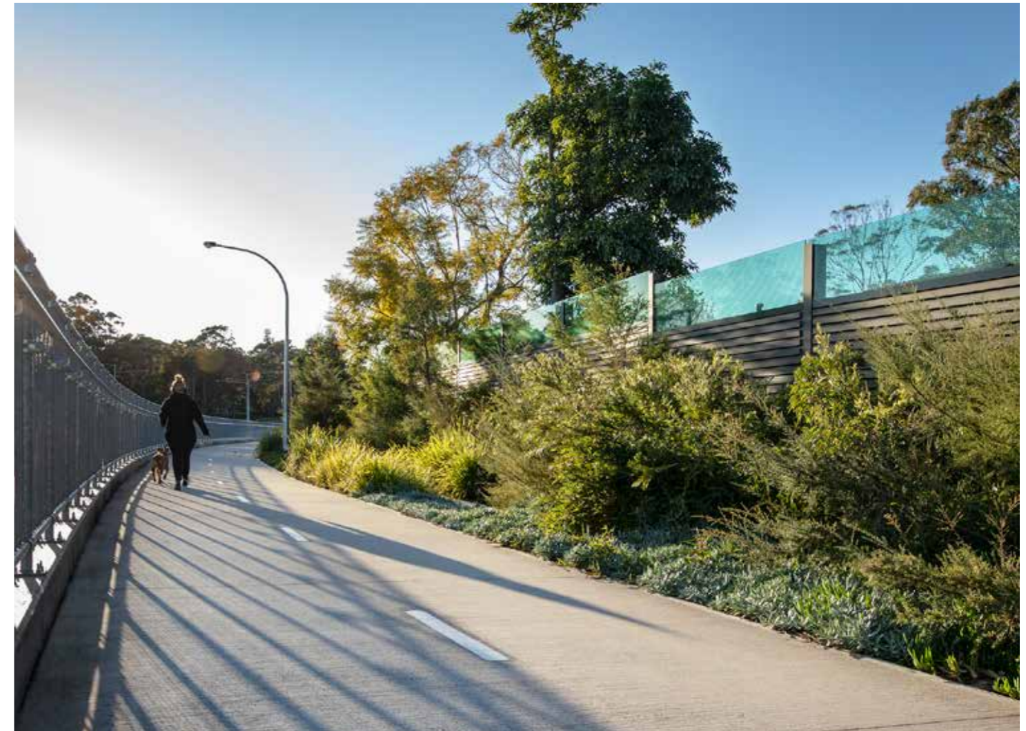
Figure 72. Northern Beaches Hospital Road Upgrade Project, Sydney. The use of planting in front of the wall softens its appearance whilst the inclusion of transparent panels reduce the visual impact of its height from the street as well as on the residential properties behind.
