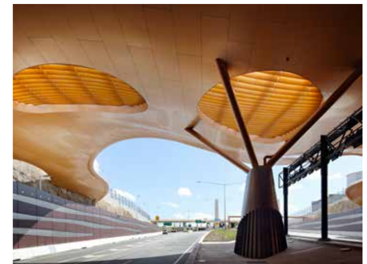
Figure 61. M7 Clem Jones Tunnel, Brisbane. The architectural solution successfully provides a distinct identity for the project.
